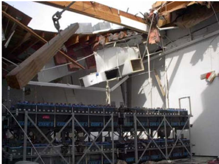
Fig. 1.1: Damage caused by the explosion in battery room in California, USA [1].
