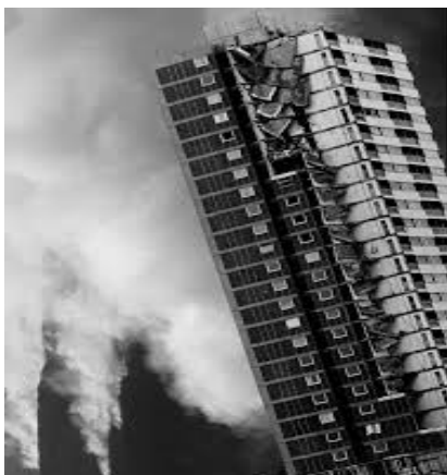
Figure 1.1: Ronan Point failure
