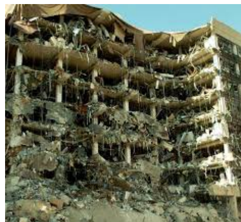
Figure 1.2: Murrah federal building failure
