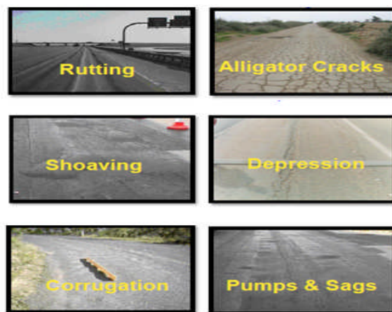
Figure 2.1 : Examples of overloading effect on roads (3)
