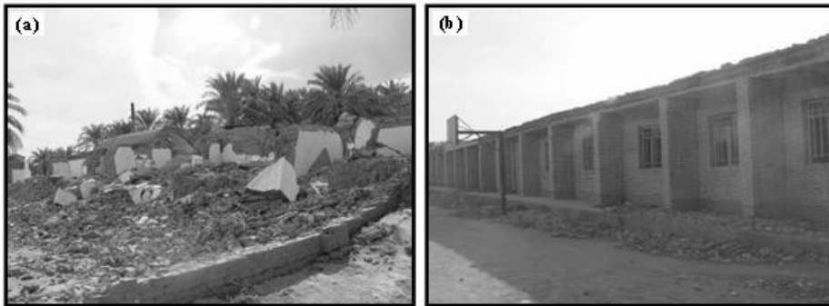
Figure 2.1: (a) A completely demolished URM dwelling, (b) An intact CM building, 2003 Bam earthquake, Iran (Eshghi and Naserasadi, 2005)
