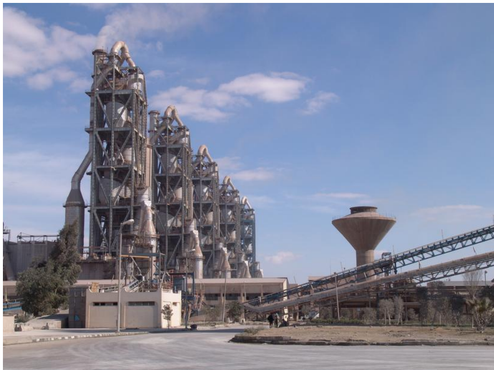
Figure (1) Lafarge Cement Egypt Plant (LCE)
