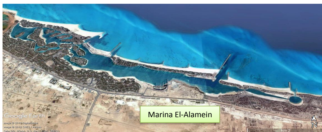
Figure (1- 3). Google satellite image showing shoreline changes at Marina El-Alamein resort
