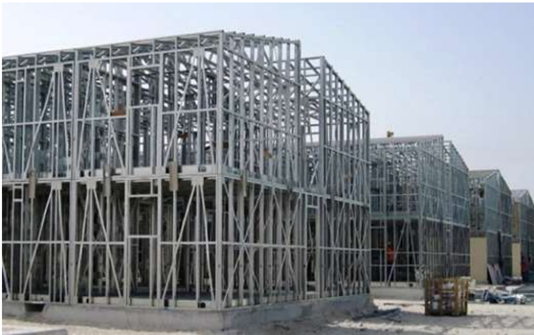
Figure 1.1 : Low rise building consists of CFS floors and walls.
