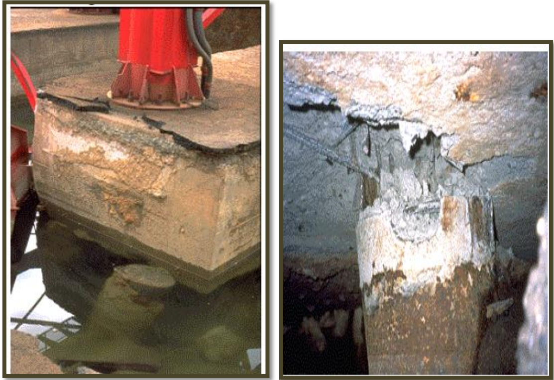
Figure 1.1 and 1.2: Detachment failures between pile head and pile cap, Higashi bridge, Hyogoken - Nanbu earthquake [1].
