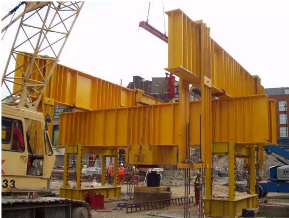
(b) Reaction frame for 30 MN reaction pile test.
